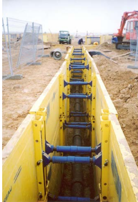
Figure 1 — Prefabricated hydraulic shoring
