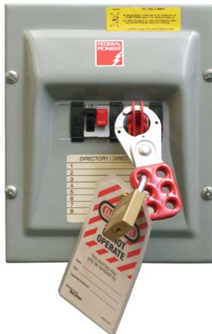
Figure 1 — Safety switch locked out
